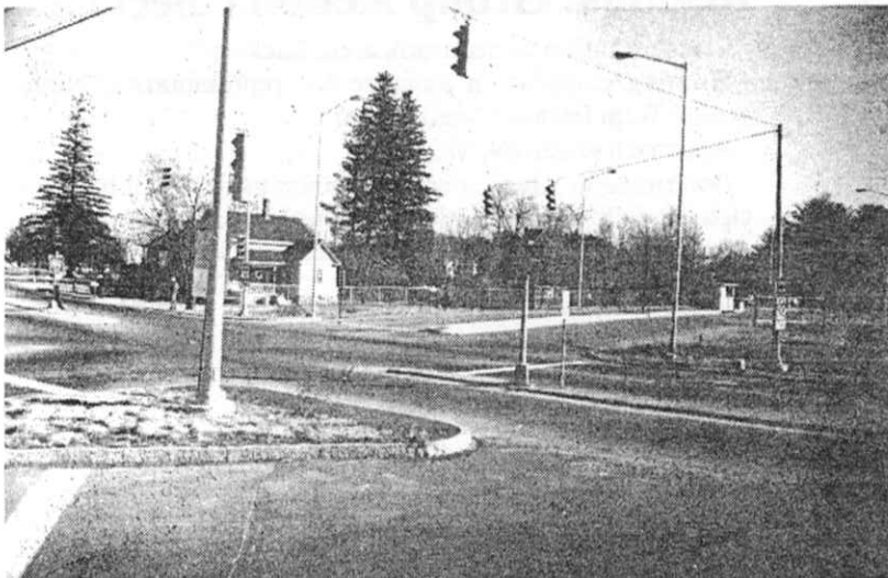
South Gate, Rts. 1 & 107 2/80
