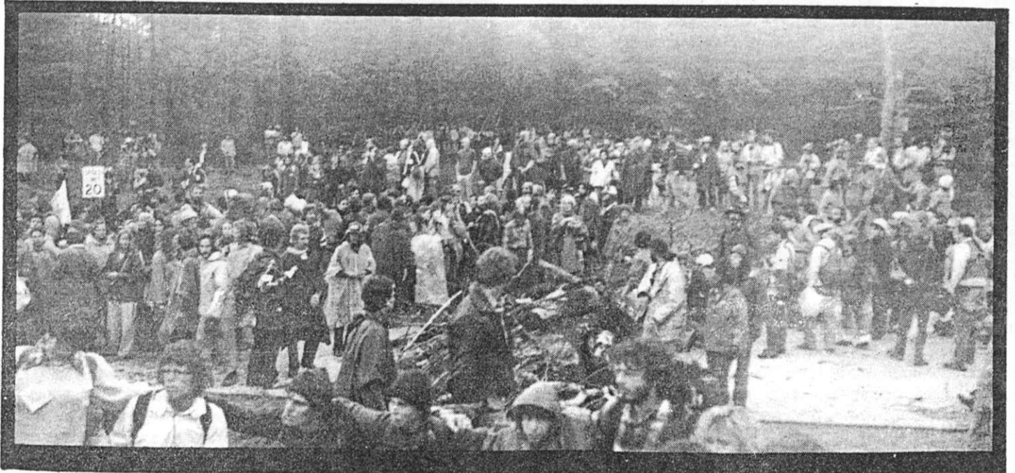
Barricades on-site on south access road 10/7/79
